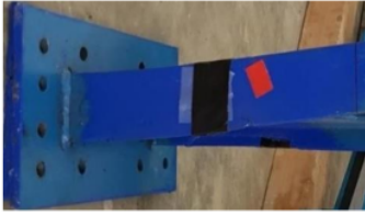
Fig. 8. Damage on WRBSC beam flange.
